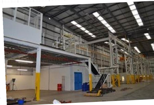
Steel Work for Mezzanine
